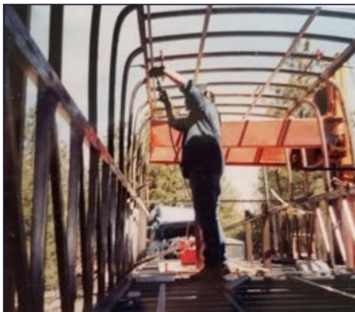
Reinforcing the girders and adding 8" to its height
