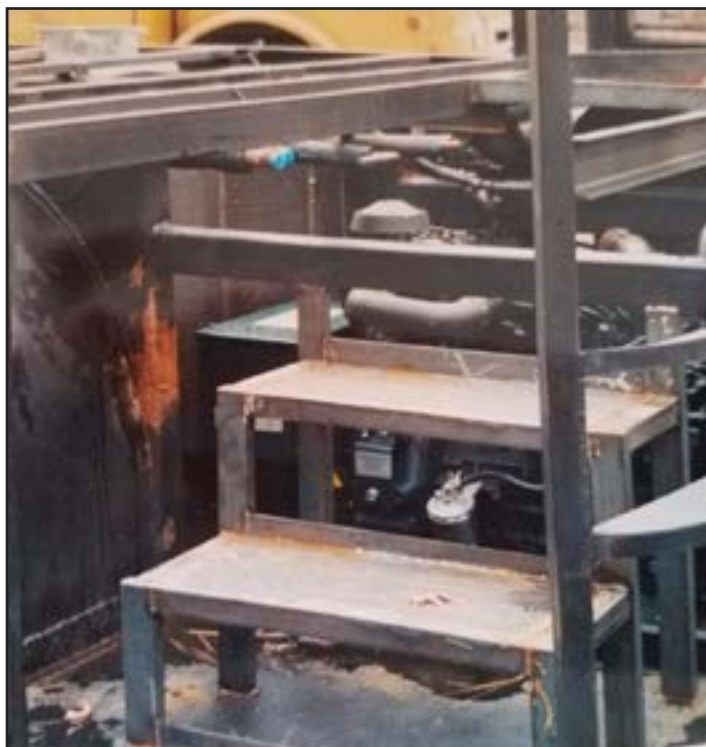
Entry Steps Construction
