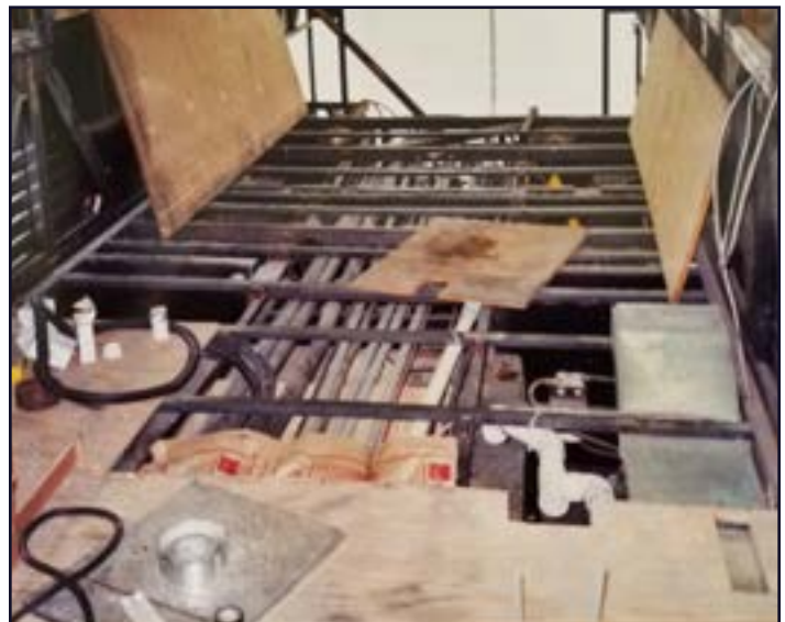
Floor was reinforced after all piping was installed
