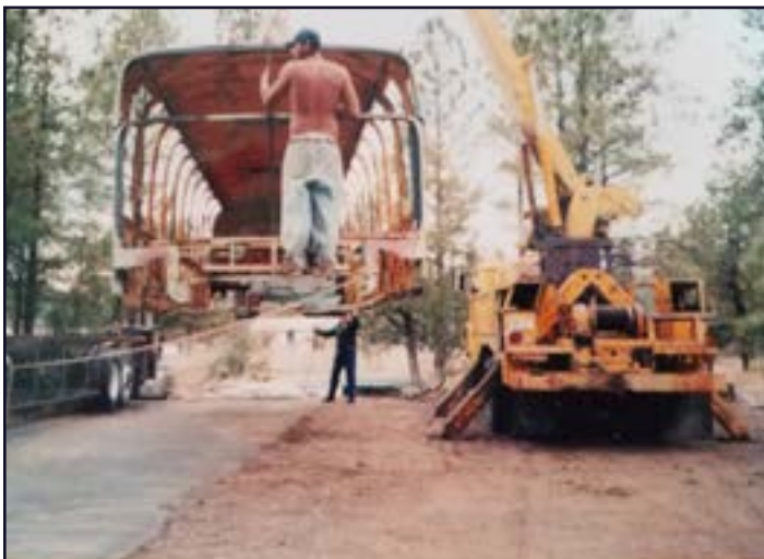
Crane lifting the top half back into place
